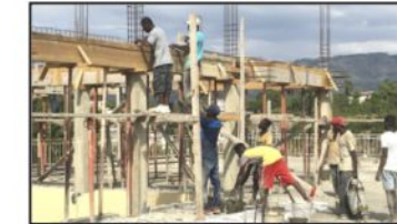
2019 Construction of new classrooms start
