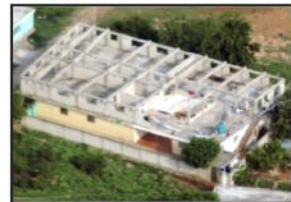
2007 School construction starts
