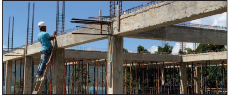
Preparing the columns for the pouring of the roof.
