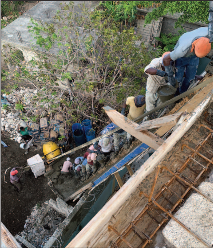
The bucket brigade moving the concrete for the roof up three stories.
